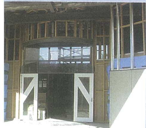
Front entrance of the sensational new art building takes shape
