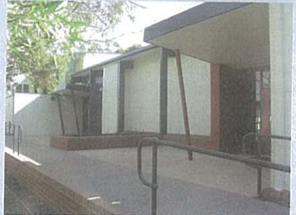
Side entrances to theatre and rehearsal rooms
